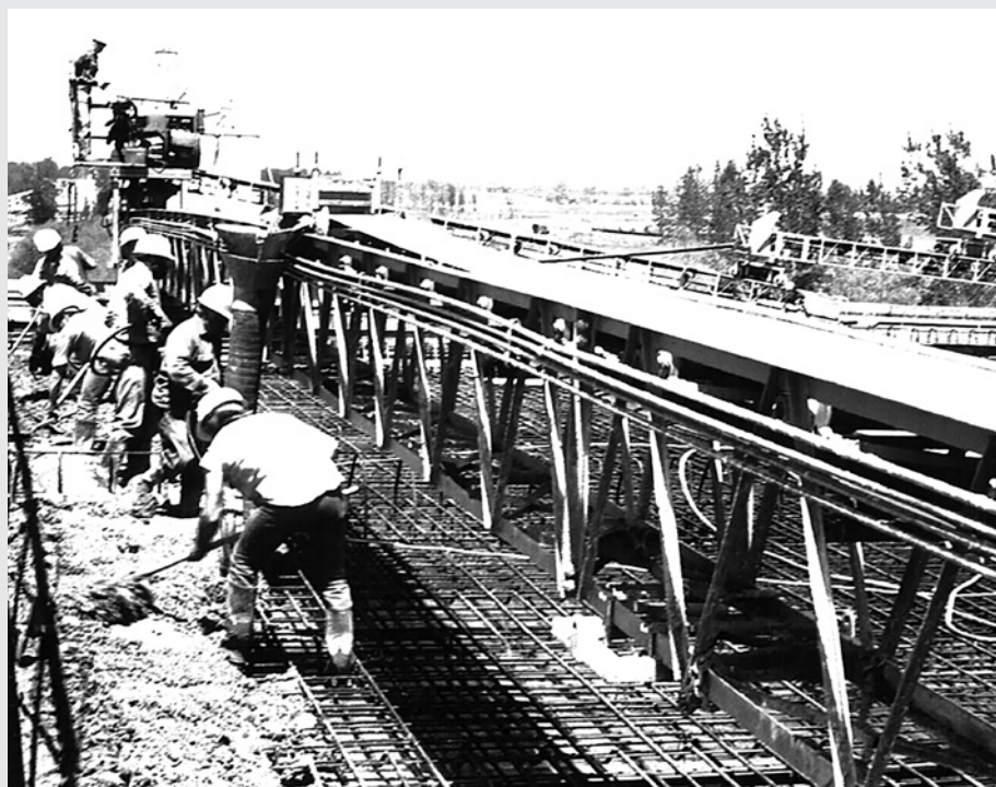
IMAGENS: GUIDE TO PLACING CONCRETE WITH BELT CONVEYORS
